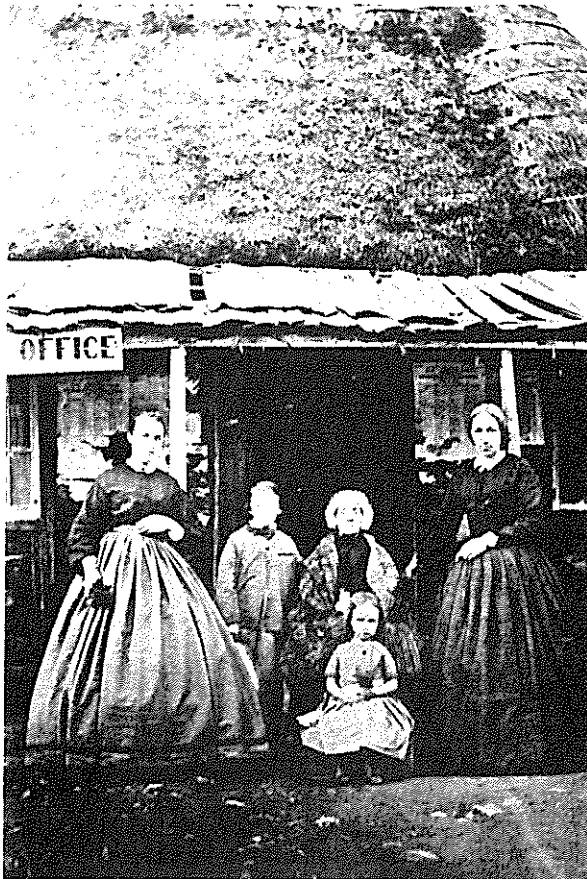
Photograph of what is thought to have been the first Kangarilla Post Office with members of the Thorpe family. Note the thatched roof, paling verandah and construction of walling by horizontal slab or drop slot technique (SA Archives)
