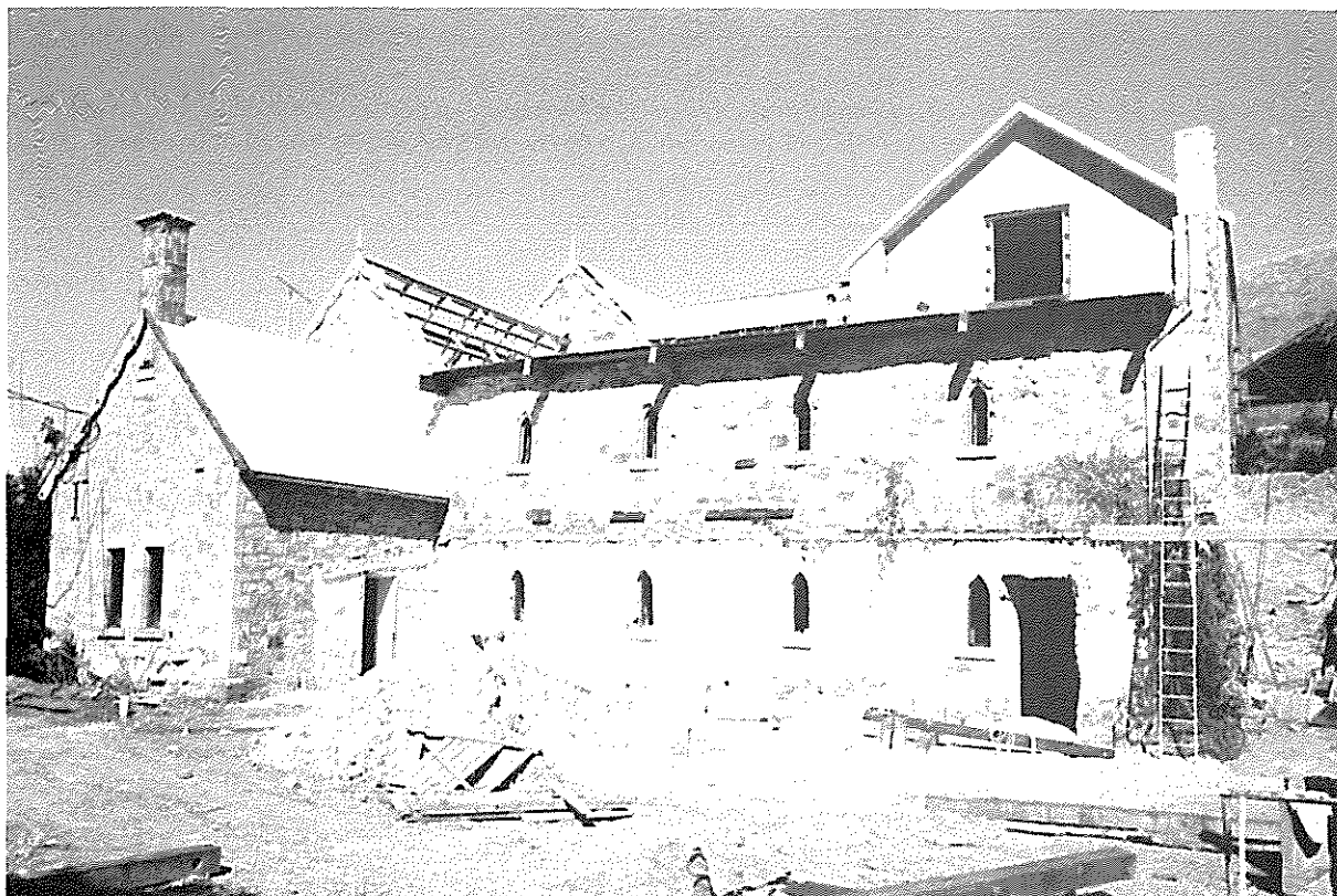
A.2.3.2 Clarendon winery, Clarendon (during renovation, 1981)
