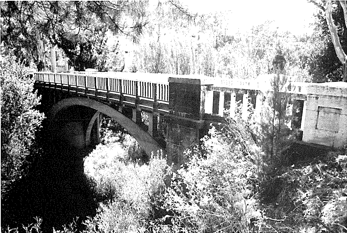
A.2.3.16 Clarendon Bridge, Clarendon
