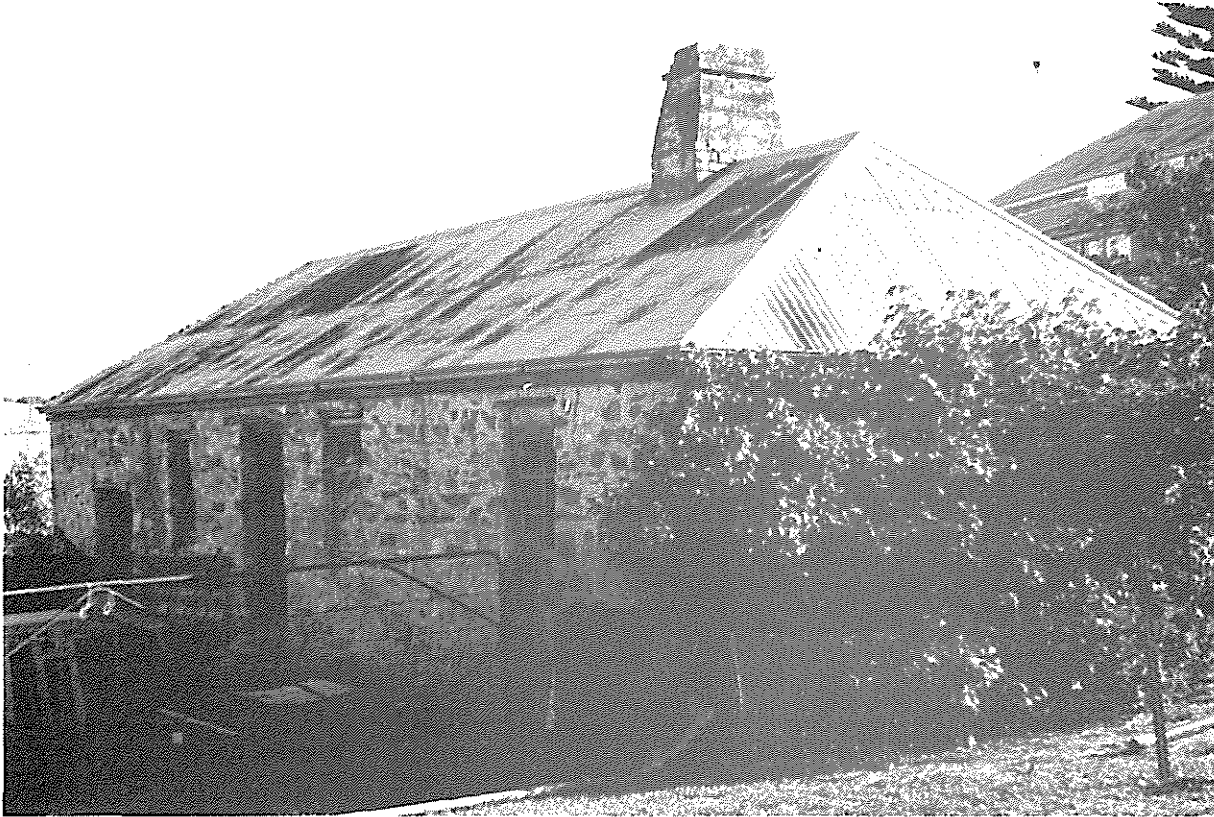
A.6.1.2 Former House Blake Road, Bull Creek
