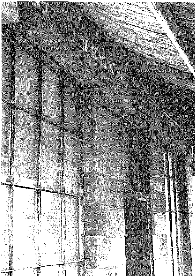
A.5.4.10 Former Store, Venables Street, Macclesfield
