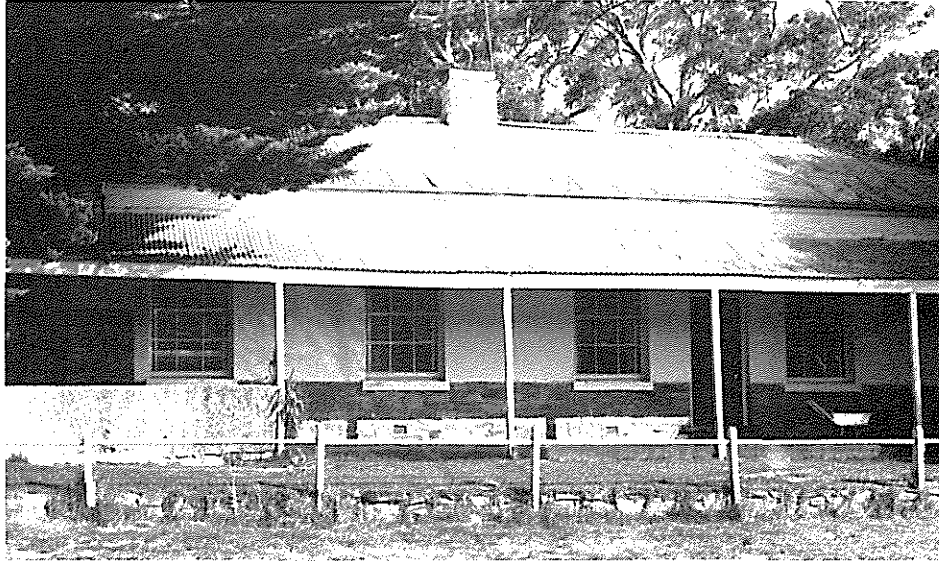
A.7.1.1 House (former Green Man Hotel), Ashbourne
