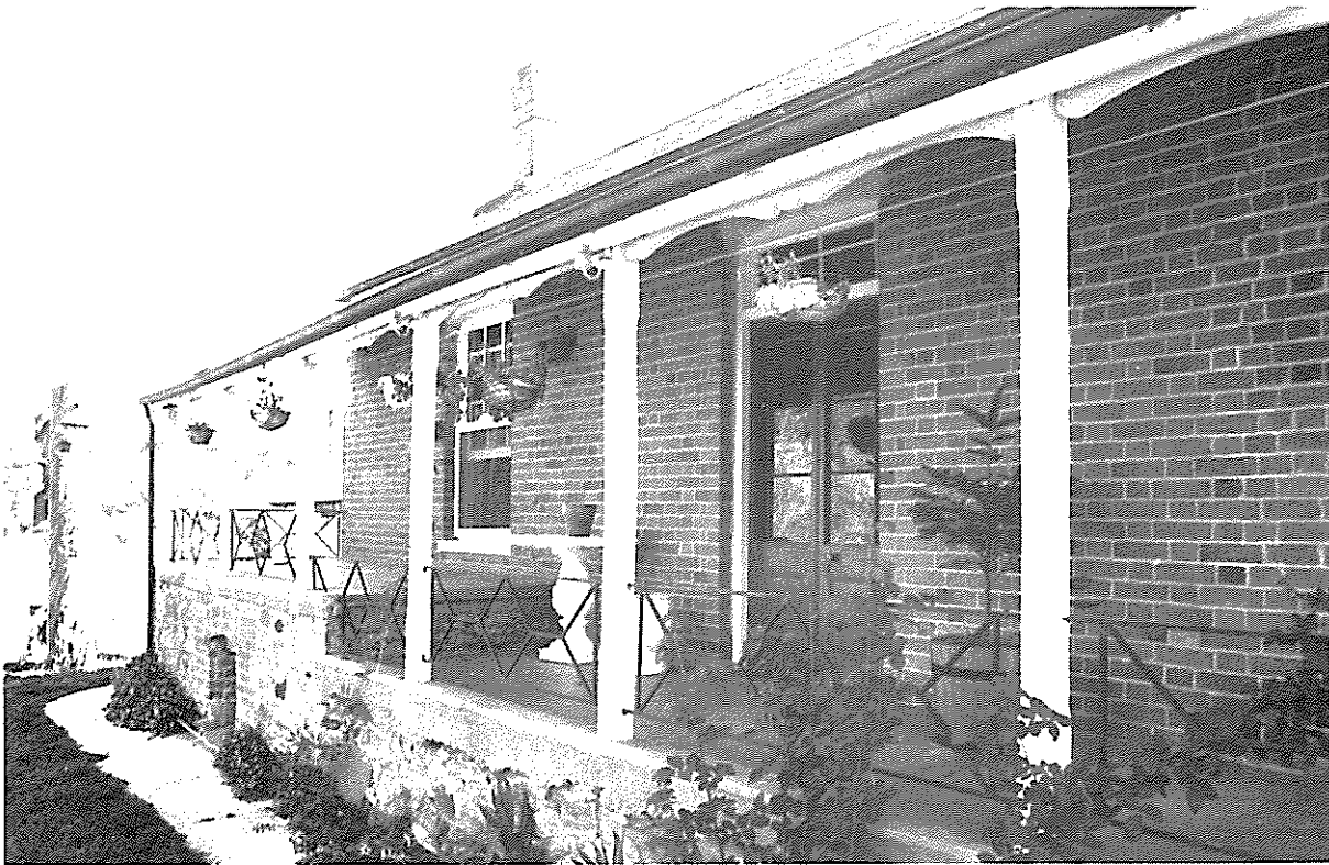
A.2.3.18 'Thrush Grove' Turners Gully Road, Clarendon
