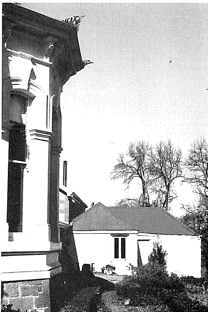
View of 'Warrakilla', part of which was known as Warland's Wheatsheaf Inn. It was later extended to become the home of G. W. Goyder, Surveyor-General of South Australia. NB This house was largely destroyed as a result of the 1983 Ash Wednesday bushfires.
