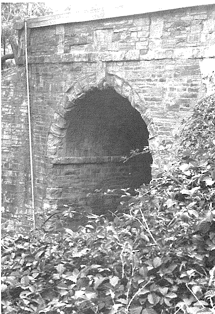
B.7.1.7 Balderson Bridge, Goolwa Road, Ashbourne
