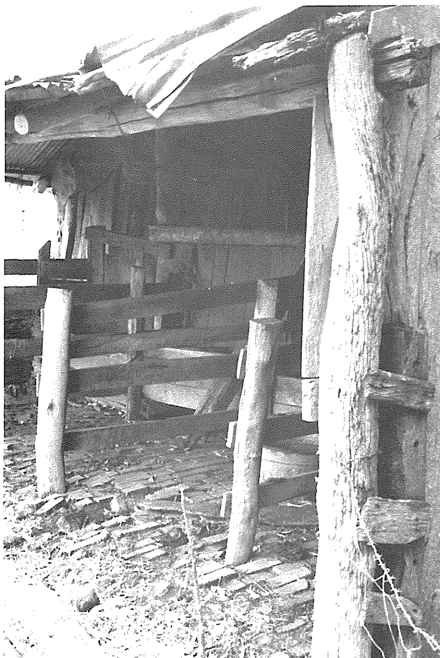
A.3.4.1 Farm building at 'Gum View' Kuitpo
