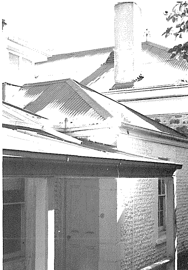
A.4.4.1 'Warrakilla' (part of which was formerly The Wheatsheaf Inn) Echunga Road, near Mylor
