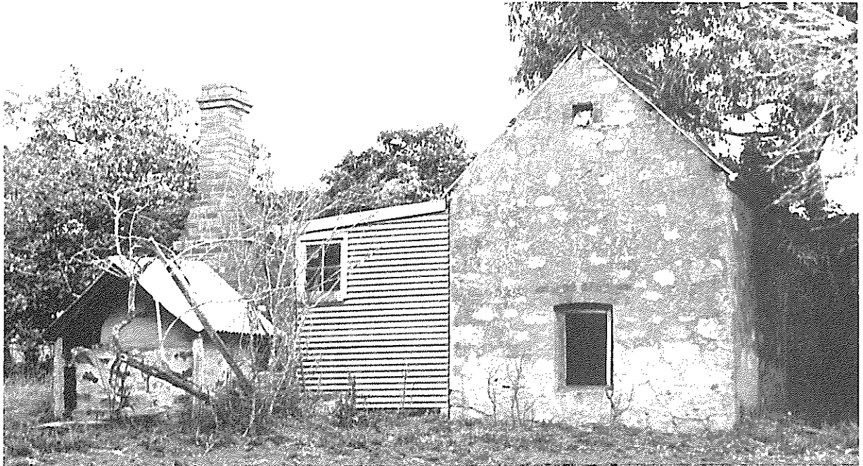
A.4.2.11 House Braendler Road, Echunga
