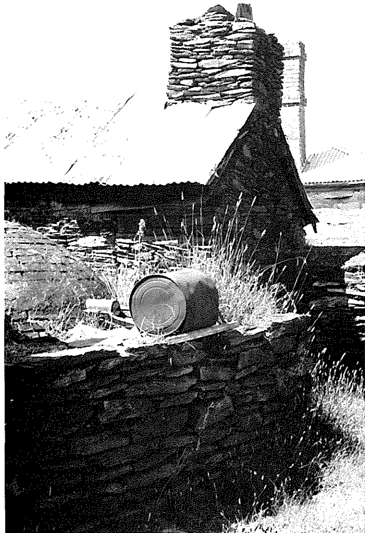
A.2.2.3 Farm Building off Hicks Hill Road Cherry Gardens
