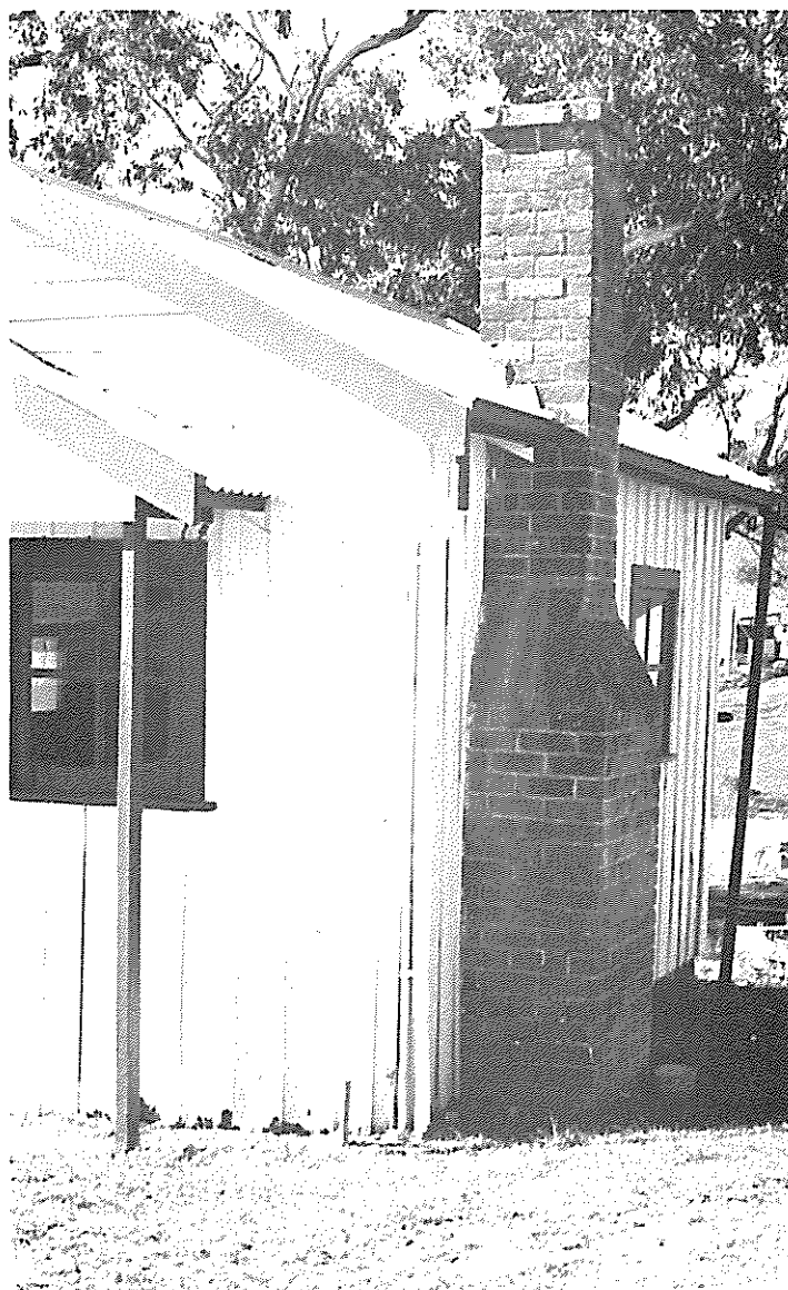
This building, the former Chapel at Kuitpo Colony, is of timber construction the form of which is largely peculiar to Kuitpo due to the proximity of local saw mills. At Kuitpo Colony this board and batten walling was complemented by more makeshift arrangements in order to house a large number of unemployed during the Great Depression.
