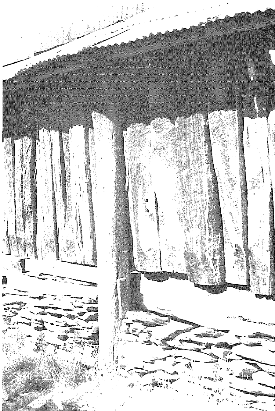
A.2.2.1 Slabshed 'Thornbury Park'
