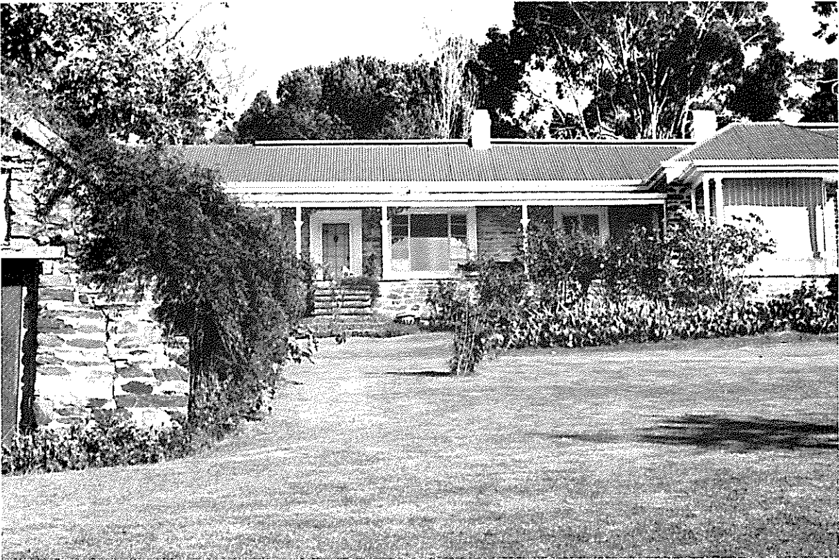
B.2.1.4 'Rockleigh' off Piggott Range Road, Angel Gully
