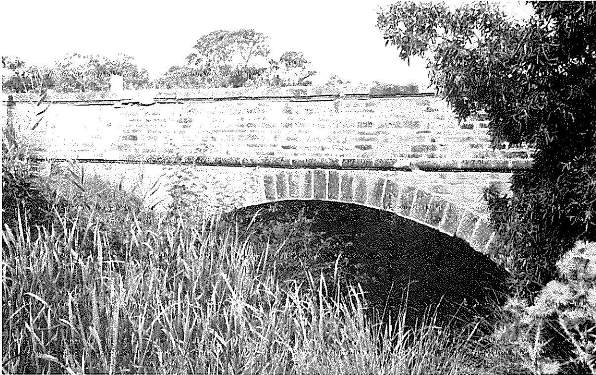
A.7.1.5 Mayfield Bridge, Ashbourne
