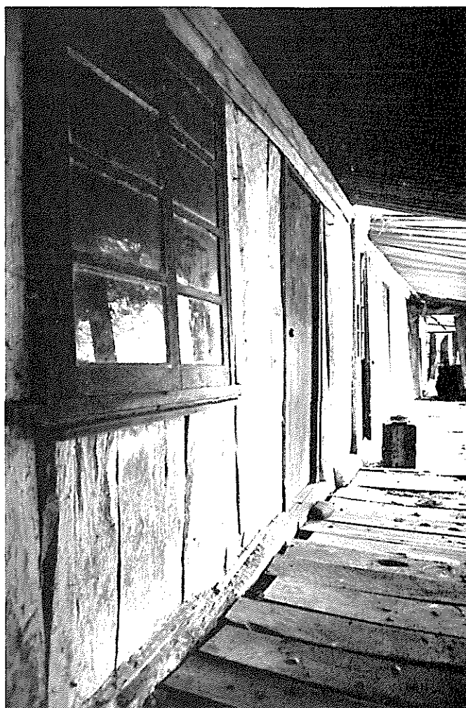
The original homestead of the Michelmore family, 'Gum View', still stands and exhibits use of both the adze and circular saw to cut and trim the locally available Red Gum
