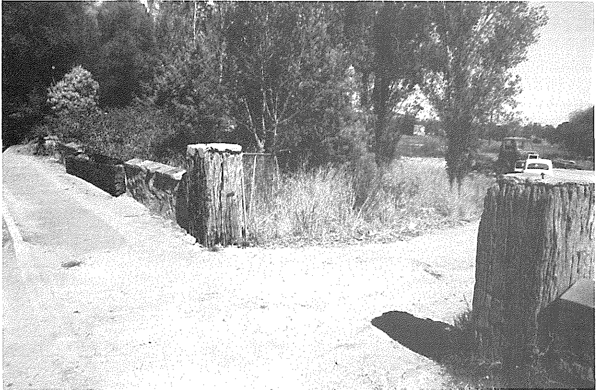
A.4.2.2 Gate Piers, Horse Trough and Well, Adelaide Road, Echunga
