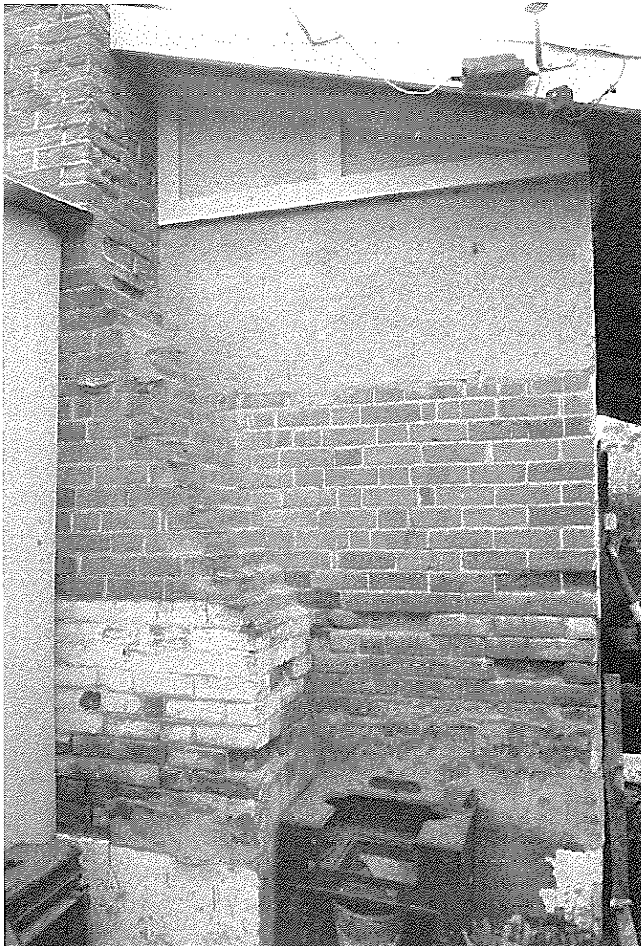
B.6.5.16 Detail of brickwork, Brookman Road, Meadows
