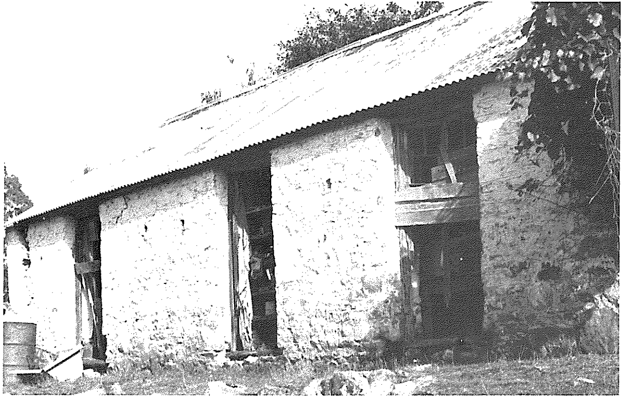
A.4.2.6 House ruins, Concannon and Sands Roads, Echunga
