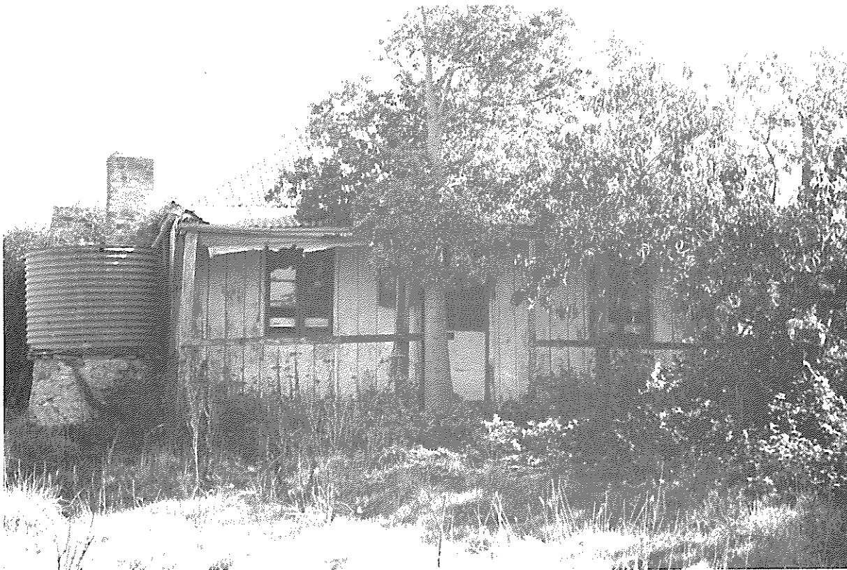
A.5.4.13 Former House, Davies Street, Macclesfield
