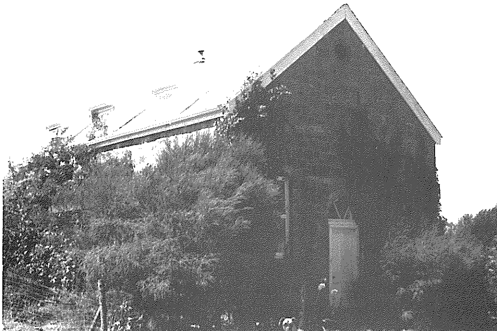
B.2.2.3 Former Rechabite Hall Hicks Hill Road, Cherry Gardens
