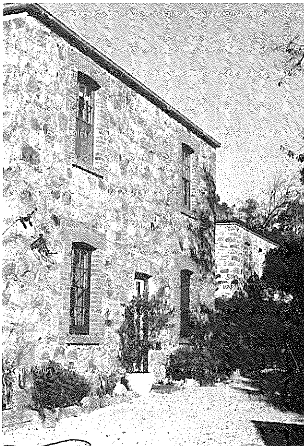
A.2.4.5 Former biscuit factory foreman's residence Main Road, Coromandel Valley
