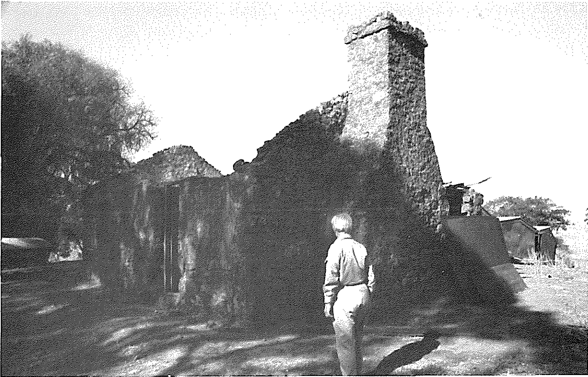
A.5.4.16 Rankine House Ruin, Strathalbyn Road, Macclesfield
