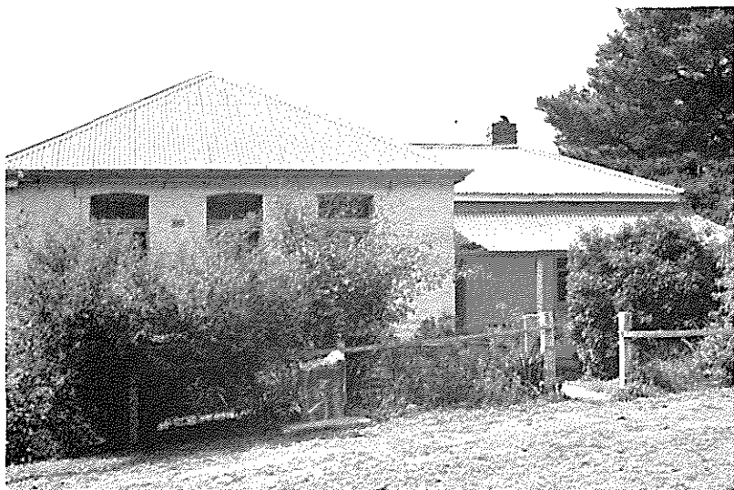
B.6.7.1 House (former school), Prospect Hill
