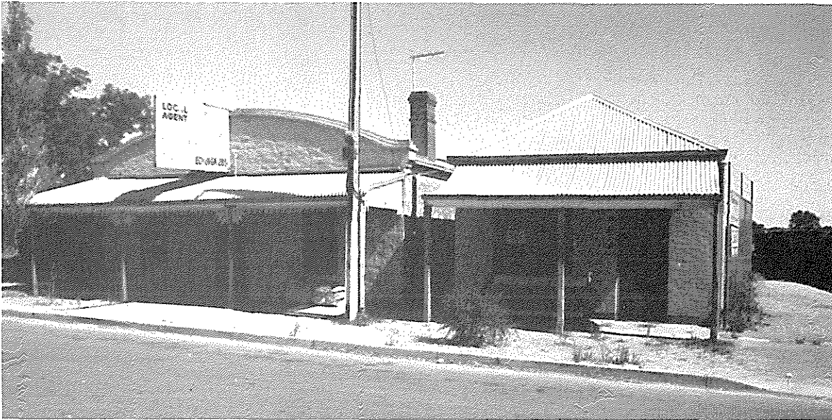
A.4.2.3 Former Coaching Station, Adelaide Road, Echunga
