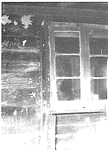
A.3.3.7 House of drop-slot construction off Peter Creek Road, near Kangarilla
