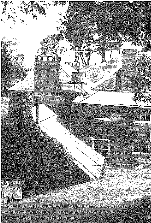
A.3.2.5 'Glengrove' off Cut Hill Road, near Kangarilla
