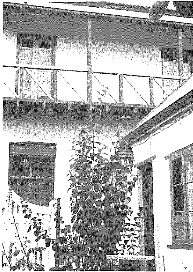
A.5.4.2 'Greenleeves Gallery', Venables Street, Macclesfield
