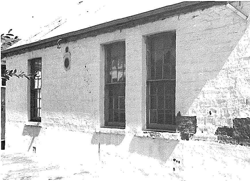
A.5.4.4 RSL Hall (former School Building), Venables Street, Macclesfield
