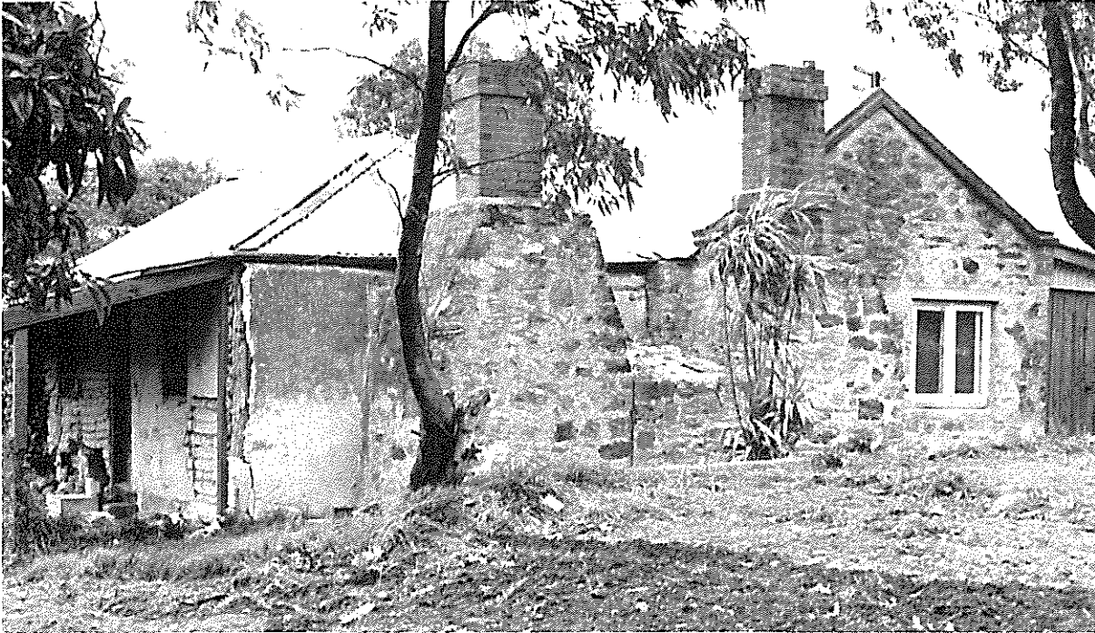
A.3.1.1 House, Baker Gully Road, Baker Gully
