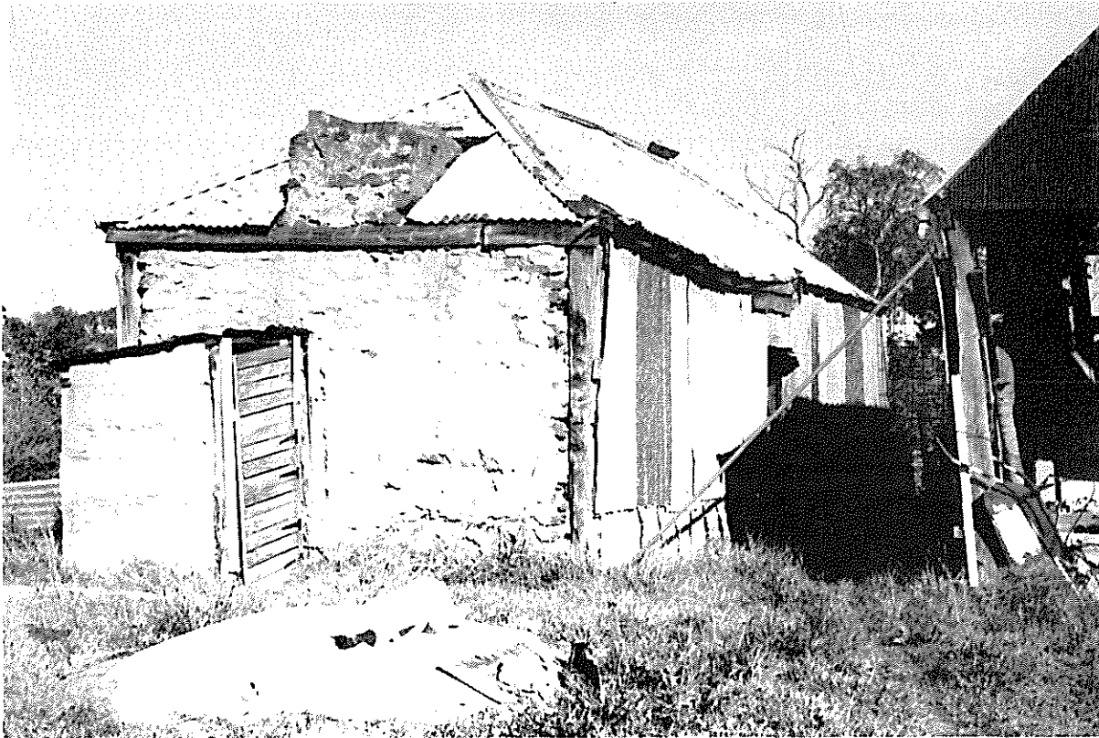
B.3.7.1 Pug outbuilding, corner Sand and Douglas Gully Road, Yarooma
